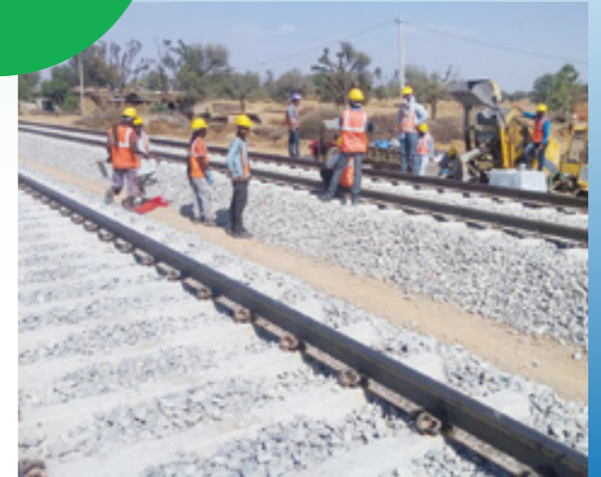
Semi-mechanised track installation
