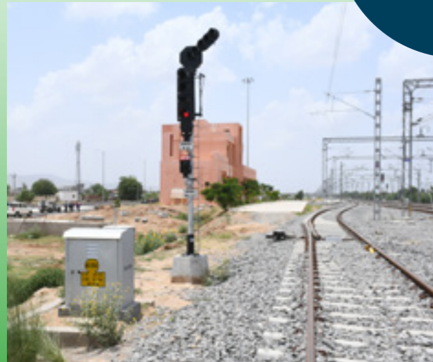
First High Rise OHE in Pipava for Kutch Railways
