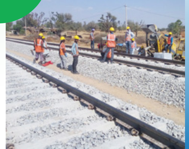
Semi-mechanised track installation
