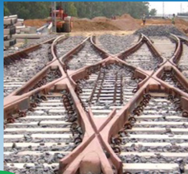
Y & D crossovers for simultaneous train receipt & dispatch
