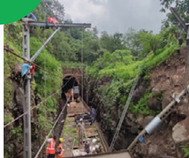
OHE Modification & replacement of Kasara & Lonavala OHR in Ghat section
