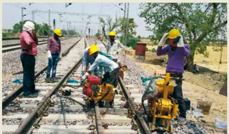
Semi-mechanised track installation
