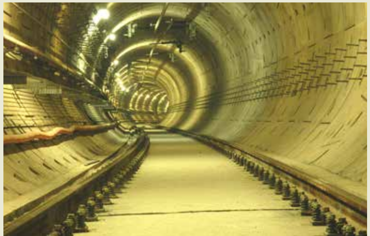
Ballast-less track in a circular tunnel
