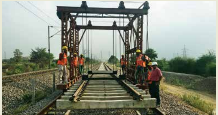
Semi-mechanised track linking
