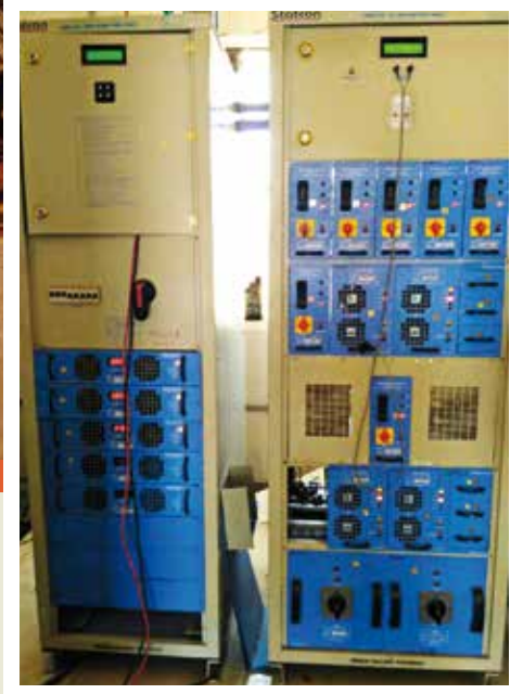
Equipment installation for indoor signaling
