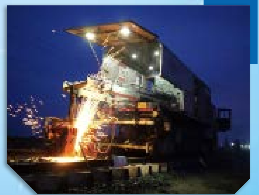
Flash Butt Welding Machine working on Eastern Dedicated Freight Corridor Project
