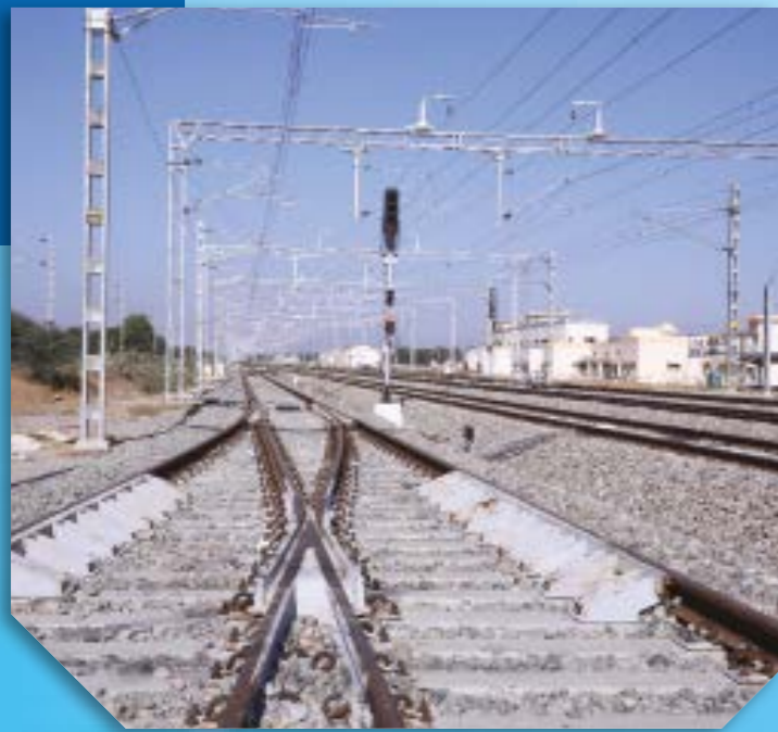
Turnout and Main Signal
