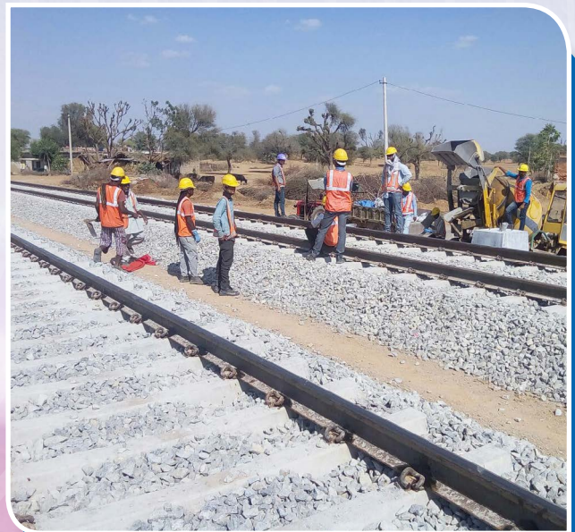
▲ Semi-mechanised track installation
