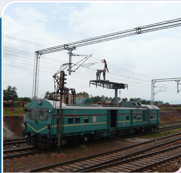
▲ High Rise OHE job in progress at Port Pipavav, Gujarat
