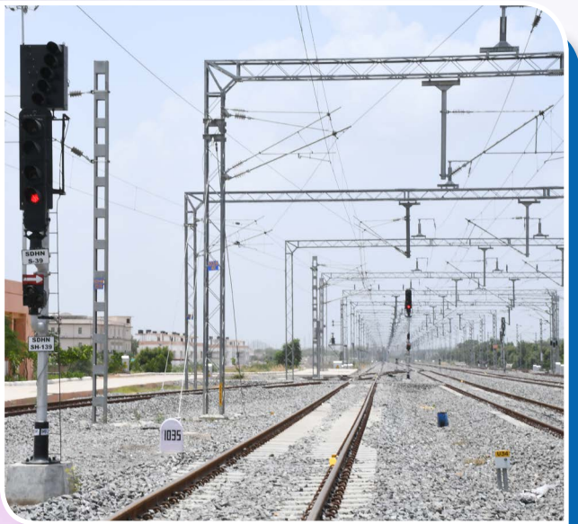
Working Signalling Gears in WDFC
