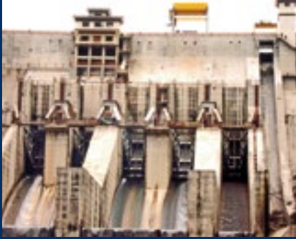
Hydro-mech Gates at Tala, Bhutan
